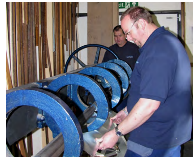
Rolling Zinc sheets to form pipes
